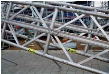
(1) Preassembly of roof girders
