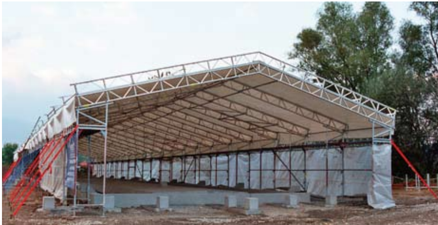
Foundation slab concrete sealing
