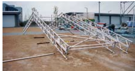
(3) Reinforcement of roof girders
