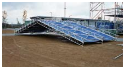
(4) Installation of rail sheets
