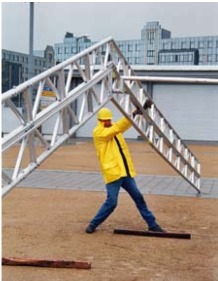
(2) Setting up of roof girders
