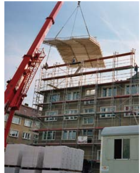
(5) Setting up the roof span
