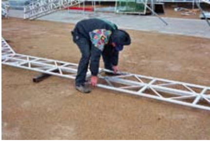
(1) Preassembly of roof girders
