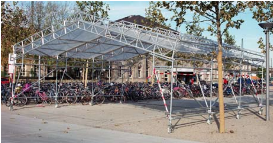
Mobile weather protection hall
